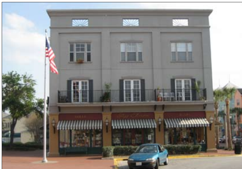
This facade has an appropriate hierarchy of windows.
