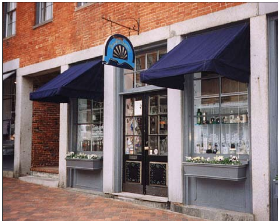
Example of canvas awnings located within building elements.
