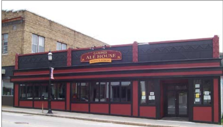
View of the recently completed facade of the Gardner Ale House
