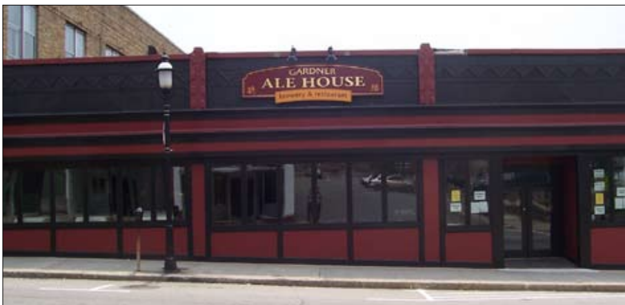
View of the recently completed facade of the Gardner Ale House
