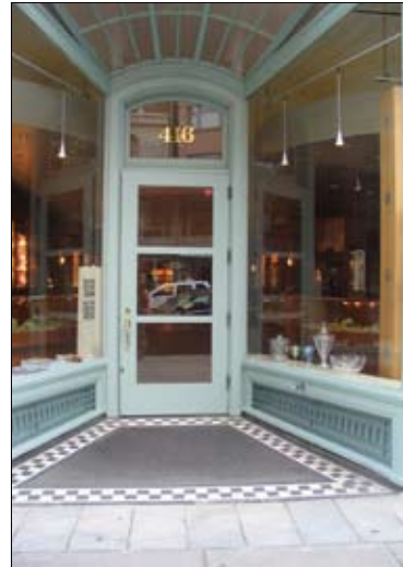
Door transoms with building address provide a legible urban environment.
