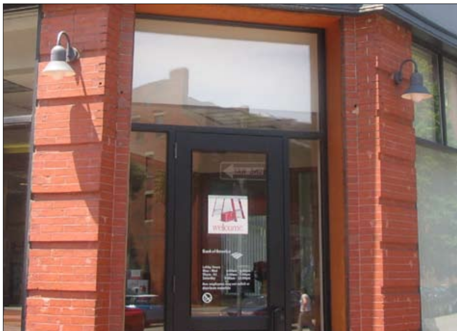
Appropriate, pedestrian-scaled lighting minimizes light pollution.
